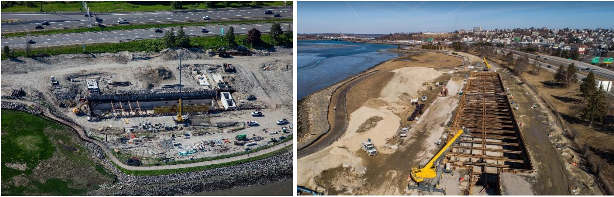
Construction of the City of Portland's Back Cove South Storage Tank Project at CSOs #017, 018, and 019 (photo credit to Maine Imaging for left side photo and Bulldog Aerials for right side photo)
