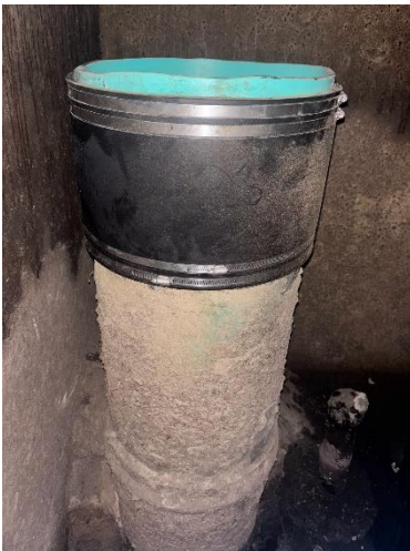
CSO regulator weir modifications at CSO #002 In Mechanic Falls (left) & CSO #002 In Winslow (right). Both weirs were raised to increase in-system storage and reduce CSO discharges
